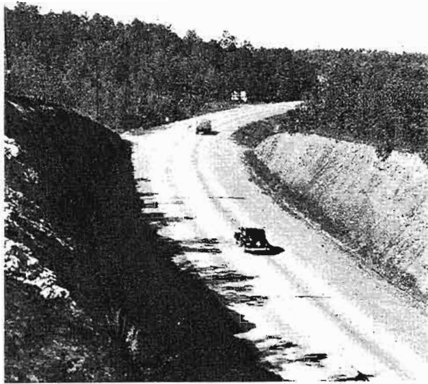
Heavy Construction on Arterial Route
