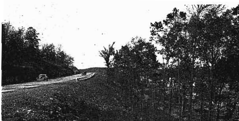
Relocation Removes Bottleneck on U. S. 64-65 Near Little Rock
