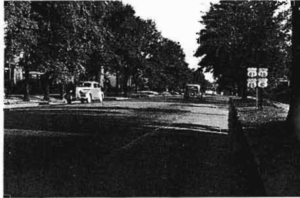
Municipal Routes are Maintained by The State
